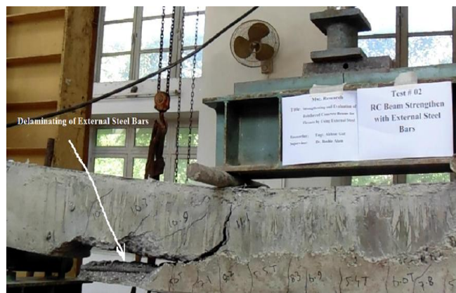
Figure: 7 Failure of Beams Strengthened with External Steel Bars
